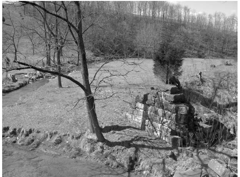
This view shows the old rail bed as it followed Crab Creek and the stone base of the bridge.
